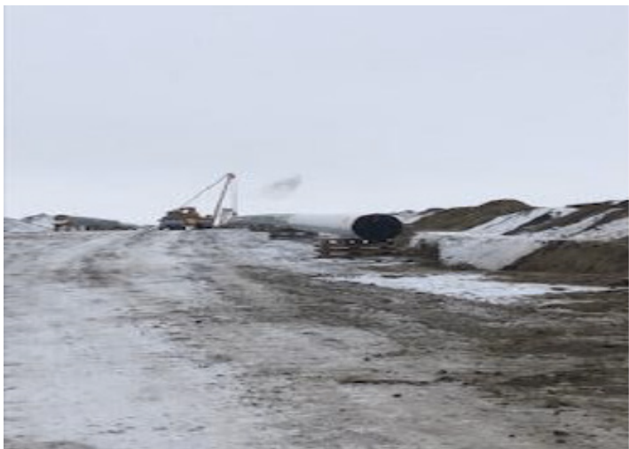
Lowering-in crew waiting on ditch – km 253+900 – Nov 19, 2018
