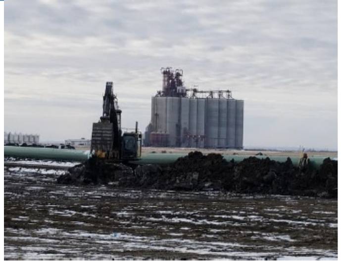
Digging ditch – km 264+350 – Nov 23, 2018
