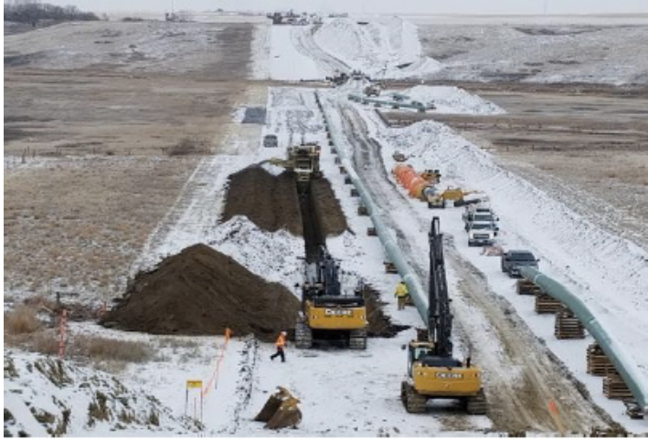
Digging ditch at heritage site - km 254+400 – Nov 19, 2018
