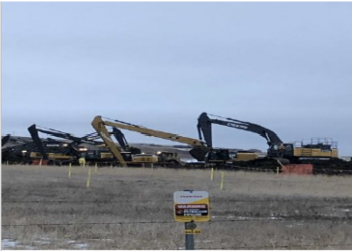
Cleaning up and backfilling – SF 141 – Nov 24, 2018
