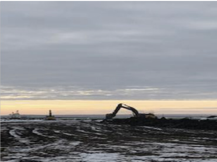
Excavators digging ditch – km 264+500 – Nov 23, 2018
