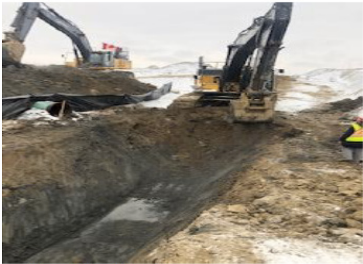
Digging tie-in ditch – km 222+670 – Nov 19, 2018
