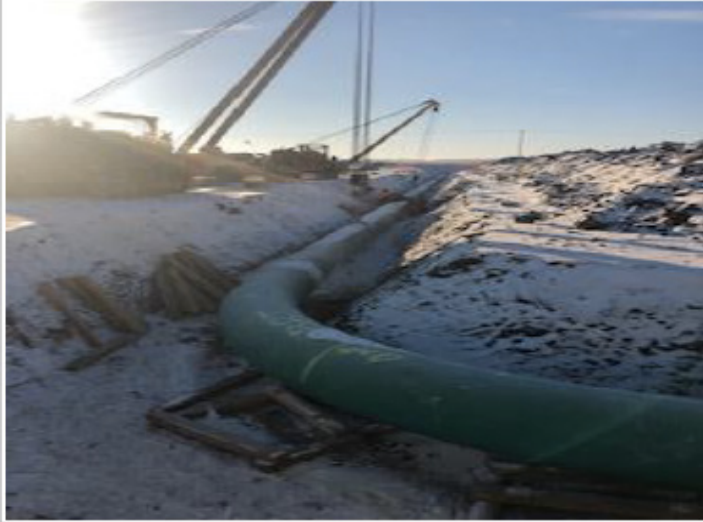
Tie-in crew weld – km 224+590 – Nov 20, 2018
