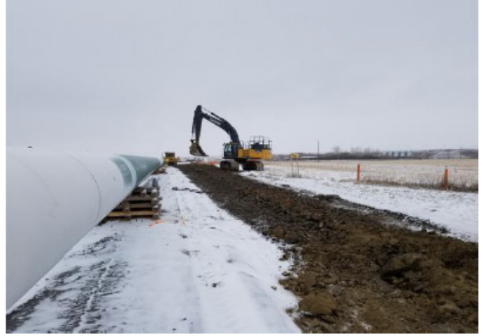
Dozer ripping frost - km 255+850 – Nov 19, 2018
