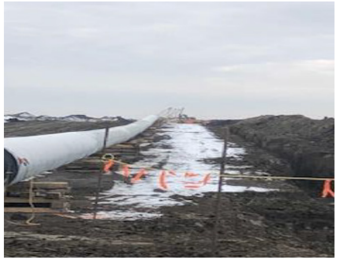
Lowering-in crew waiting on ditch – km 263+800 – Nov 23, 2018
