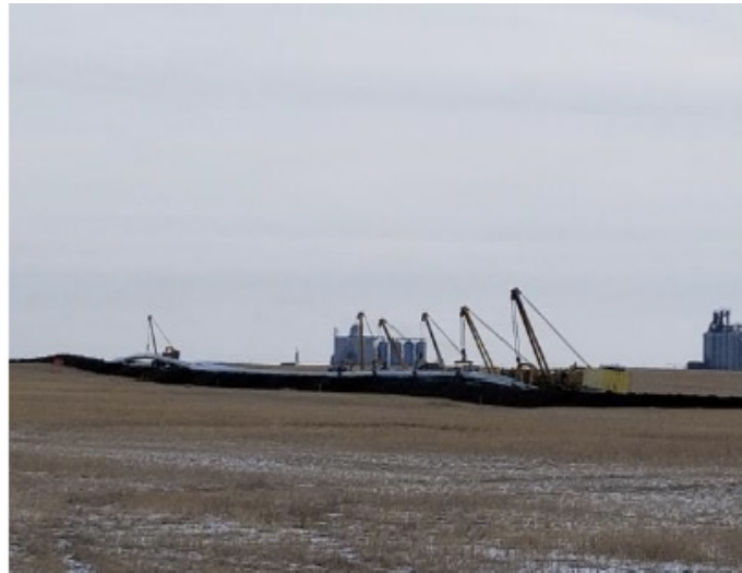
Lowering in pipe – km 262+631 – Nov 22, 2018
