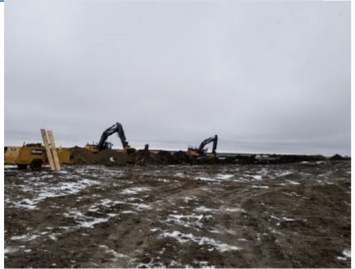
Backfill– km 264+550– Nov 24, 2018
