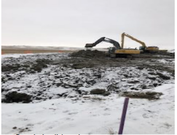
Tie-in backfill excavator in Stranraer Valley– Nov 19, 2018
