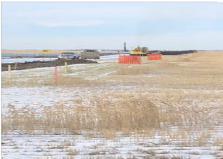
Ditching wheel working – km 262+800 – Nov 22, 2018
