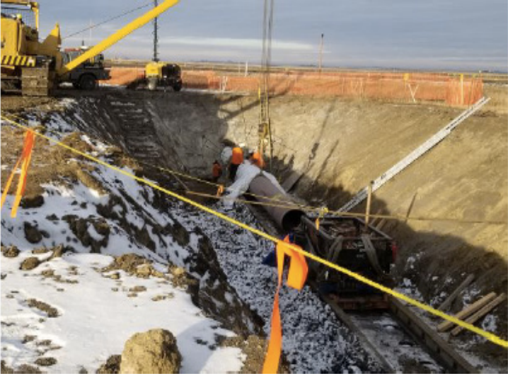
Track bore – km 266+700 – Nov 23, 2018
