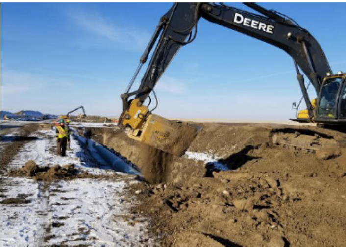
Shading pipe – km 254+000 – Nov 20, 2018
