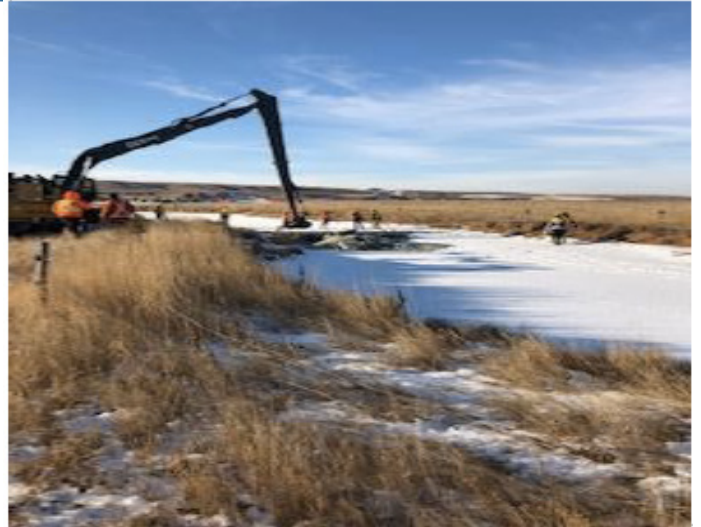
Excavator taking out ice at Eagle Creek – Nov 20, 2018
