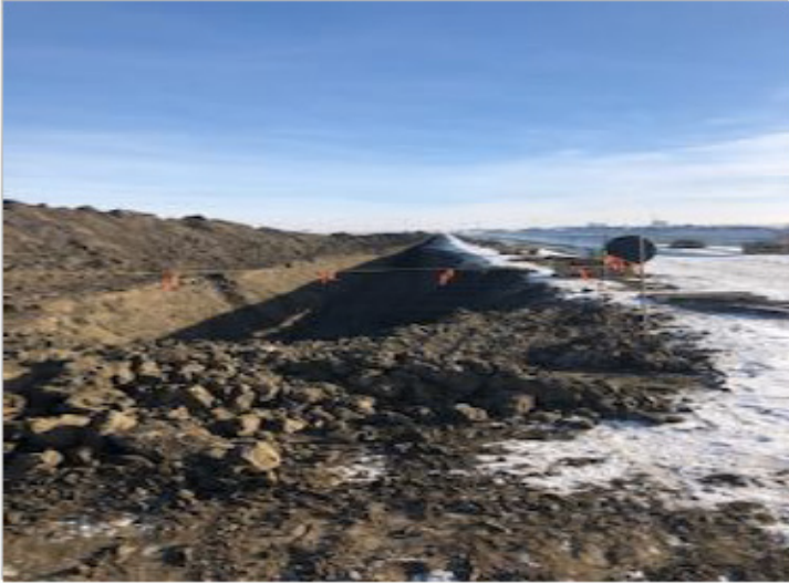
Mainline section ready for lowering in – km 260+300 – Nov 21, 2018
