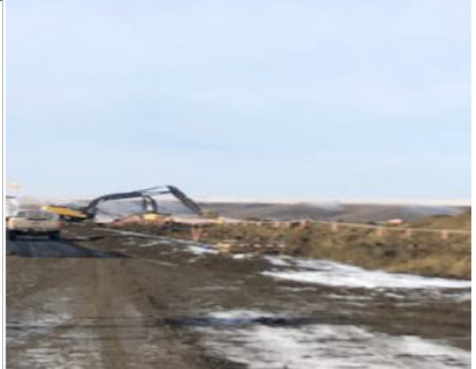
Excavator shading pipe – 255+625 – Nov 21, 2018
