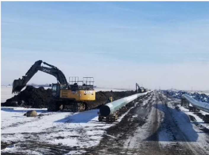
Digging ditch – km 259+300 – Nov 21, 2018
