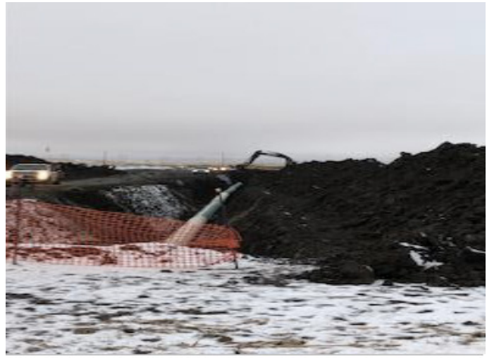
Excavator shading backfill – km 195+500 – Nov 24, 2018
