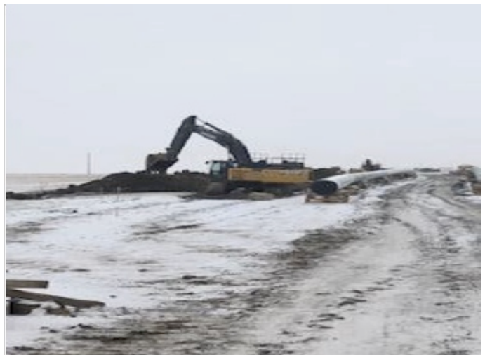
Excavator plugging out mainline– km 255+900 – Nov 19, 2018
