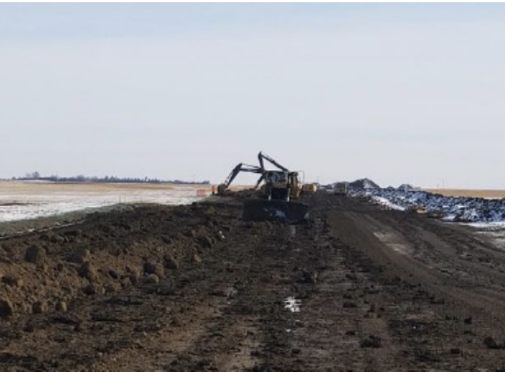
Backfill ditch – km 258+000 – Nov 22, 2018
