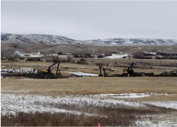
Backfilling creek section – km 222+300 – Nov 24, 2018
