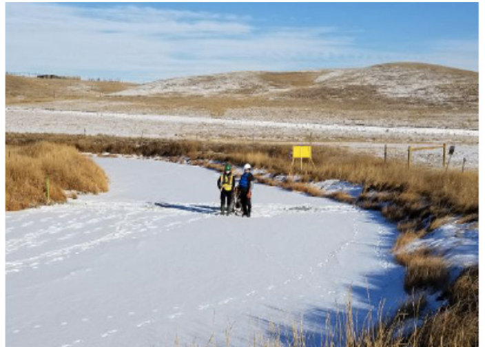
Checking water flow – km 222+100 – Nov 20, 2018
